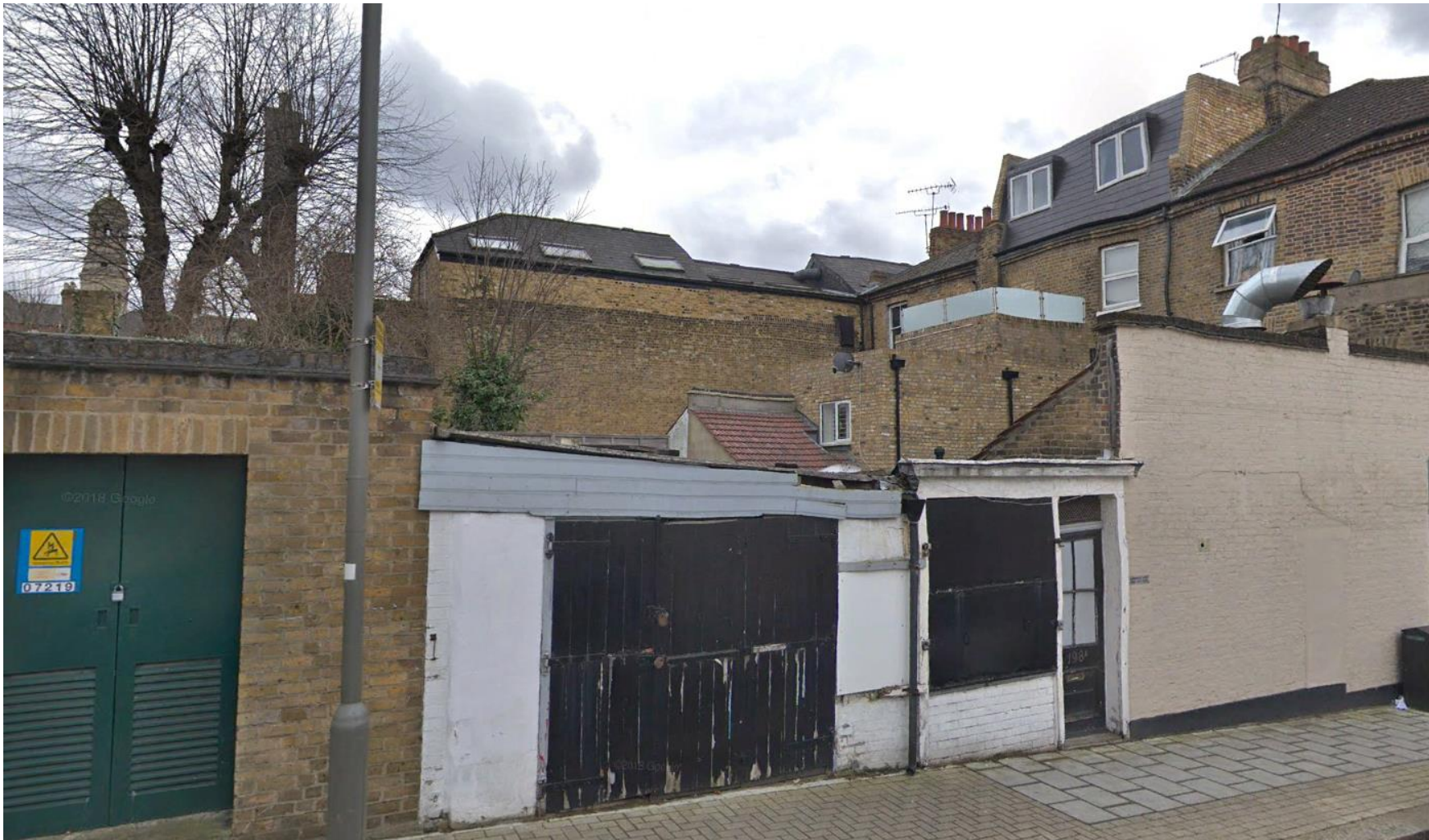
Plate 15: View of the rear from Ridgmount Road (facing SE).
